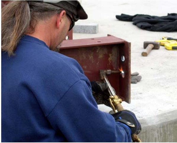
A worker enlarges anchor holes on the transmitter building support beams.
