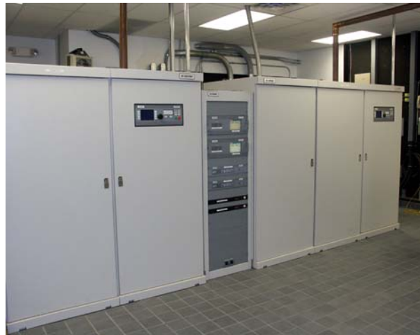
The WOR twin Harris 3DX50 transmitters, with HD rack in between.
