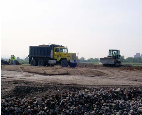
Dump trucks bringing fill material to the WOR property.
