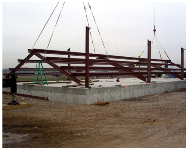
The roof trusses ready to be hoisted into place.
