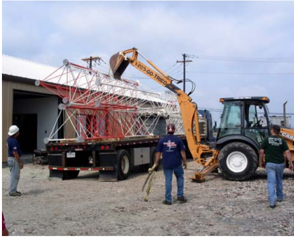
Workers from Northeast Towers remove sections of tower 2 from the delivery truck.
