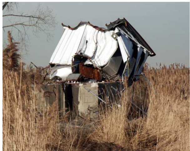
Lyndhurst tuning house 1 was hit by guy wires. The other two tuning houses survived without a scratch.
